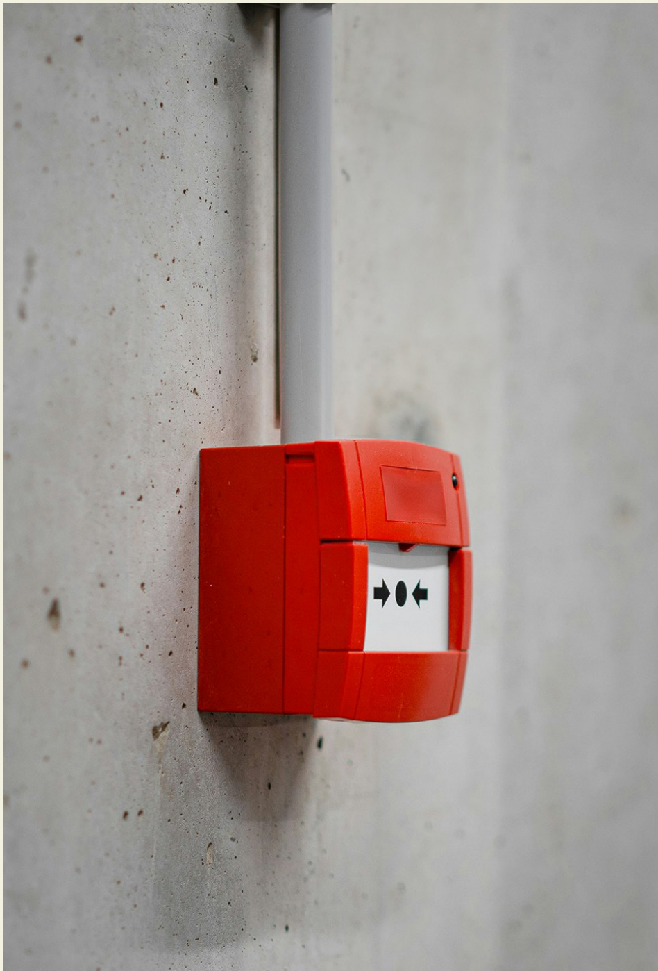
Safe fire exits
